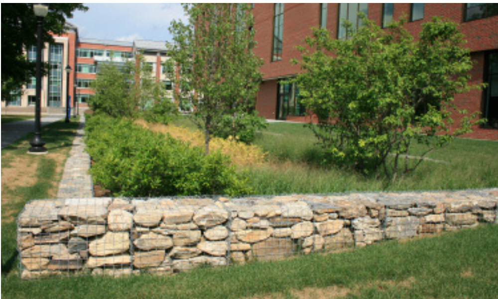
LID practices on the University of Connecticut Storrs campus. (Above 1) the pervious asphalt lot at the Towers apartment complex absorbs water during a storm. (Above 2) the green roof at Laurel Hall. (Left) the large bioretention cell next to Laurel Hall receives runoff from the non-green portion of the roof.
