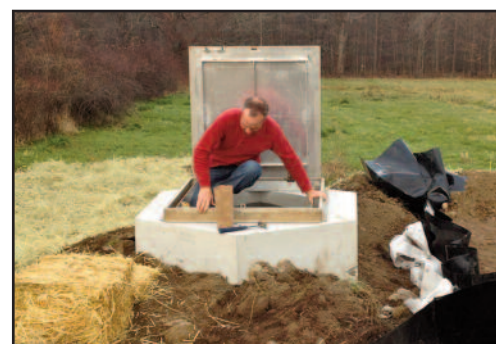
(Top) Screen capture from N-Sink in the Niantic, CT watershed. From the user-chosen location (red dot), N-Sink creates a flow path to the outlet and estimates N removal. (Bottom) NEMO’s Mike Dietz emerges from the instrument bunker used to monitor his new experimental rain garden. True to form, there were 6 more weeks of winter after this picture was taken.
